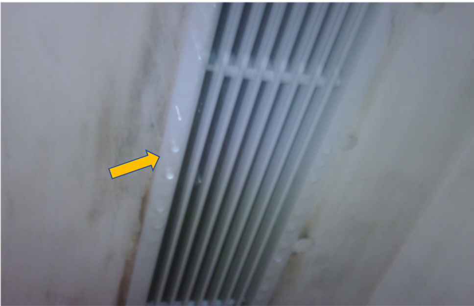
Figure 2.2a: Condensate on air diffuser surface
