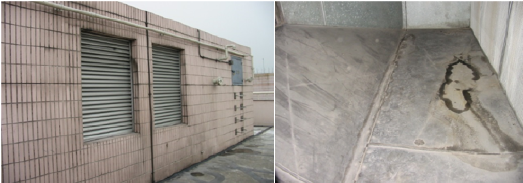
Fig. 2.3b: Poor design of architecture plenum of outdoor air intake leading to accumulation of water behind the louver
