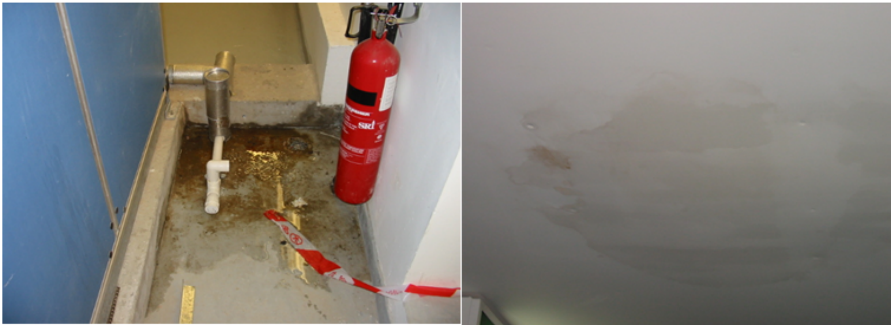
Fig. 2.3a: Active water leakage in Air Handling Unit (AHU) room and the wet ceiling below the AHU room
