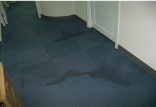
Fig. 2.3c: Water stained carpet due to past water damage
