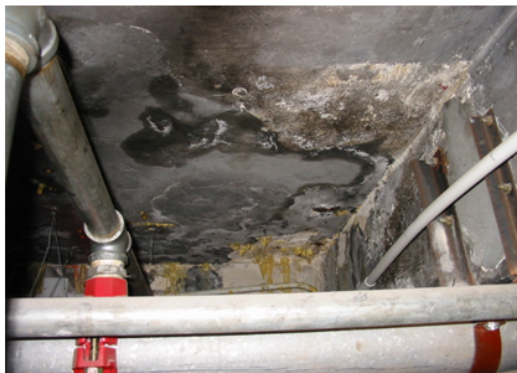
Fig. 2.3d: Water damaged ceiling in the ceiling void due to flooding in upper floor in the past
