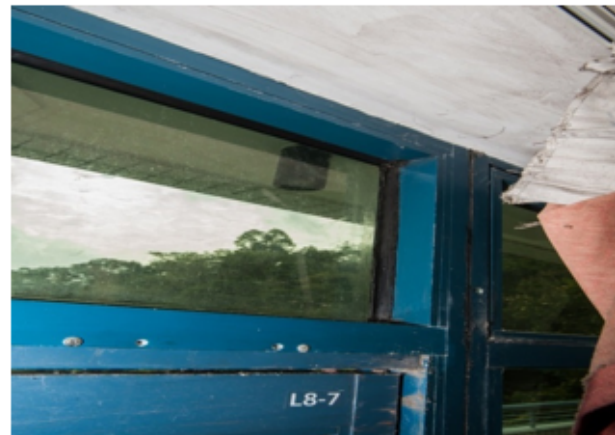
Fig. 2.3e: Past water damage on ceiling next to an improperly sealed door
