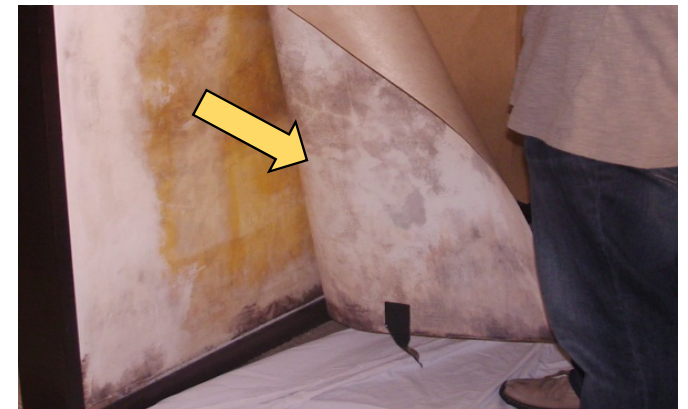
Mould growth behind wall paper
