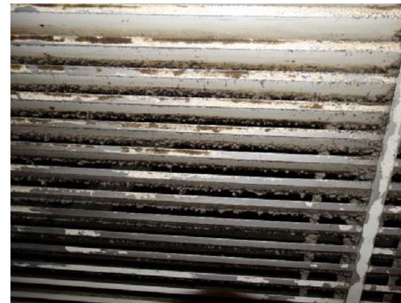
Dust (and probably mould growth ) accumulated on the surface of the air diffuser
