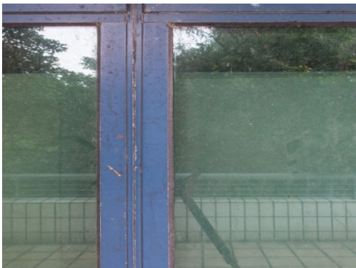
Figure 2.1d: Mould growth on aluminum window frame
