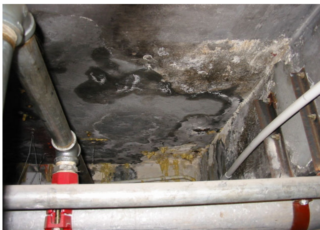
Figure 2.3d: Water damaged ceiling in the ceiling void due to flooding in upper floor in the past
